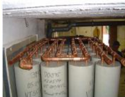
PowerTank latent heat cells are connected to a storage according to Tichelmann.
